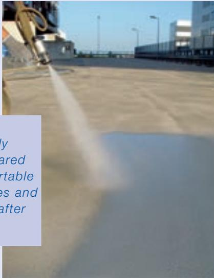
*Elastocoat is applied directly onto the prepared surface by portable spray machines and is accessible after short time.*
